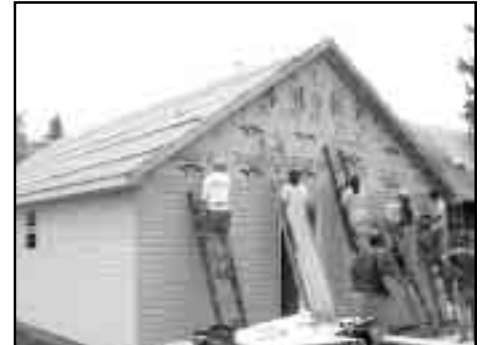
Putting up the siding.
