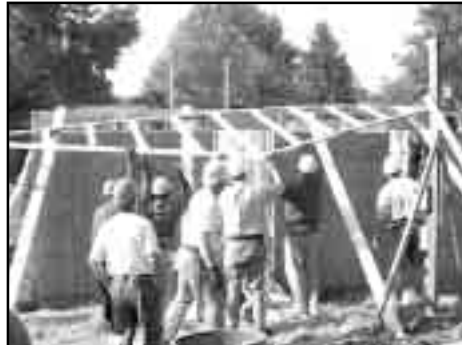
Putting up the roof trusses.
