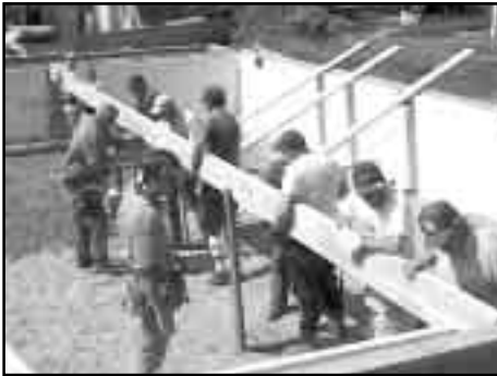
Installing the beam to lay the deck.
